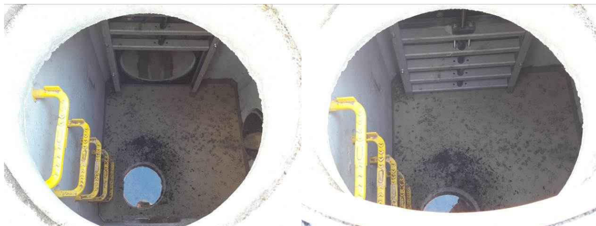
Vanne de confinement parking
